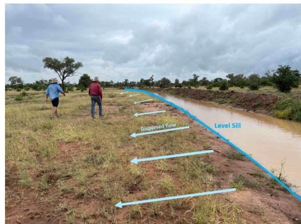
Figure 1. Level sill on water spreading structure.
